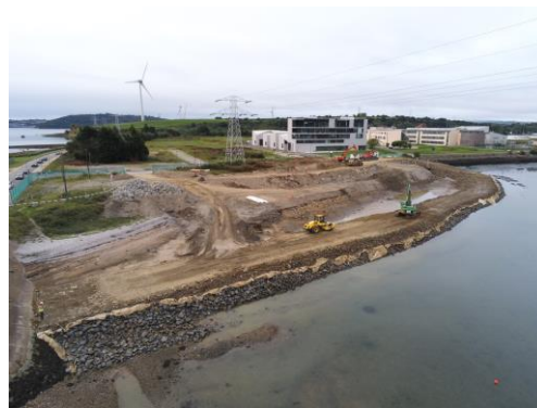
Revetment Construction
